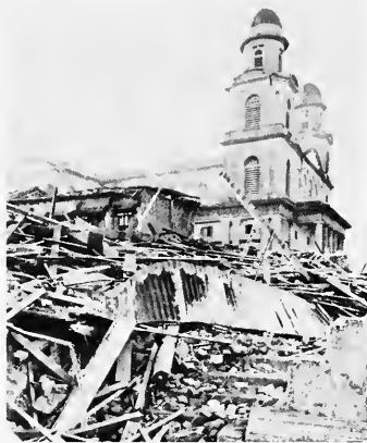
Managua church stands intact amid ruins
